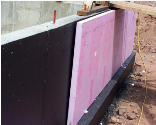
Exterior insulation R-10 continuous
