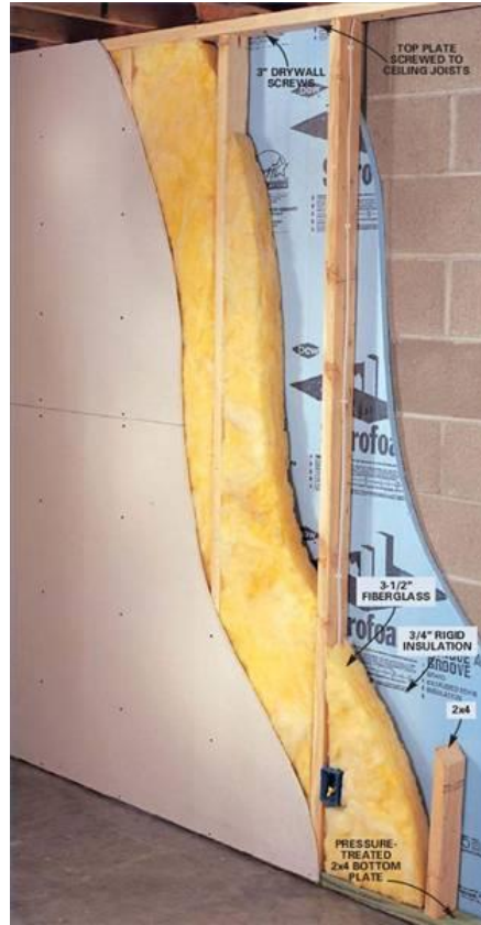
Recommended wall assembly. R-13 batt applied over R-5 foam. This is equivalent to an R-21 wall.
