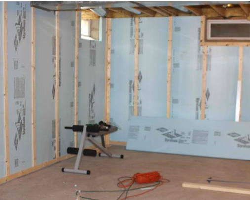
Interior insulation R-15 continuous
