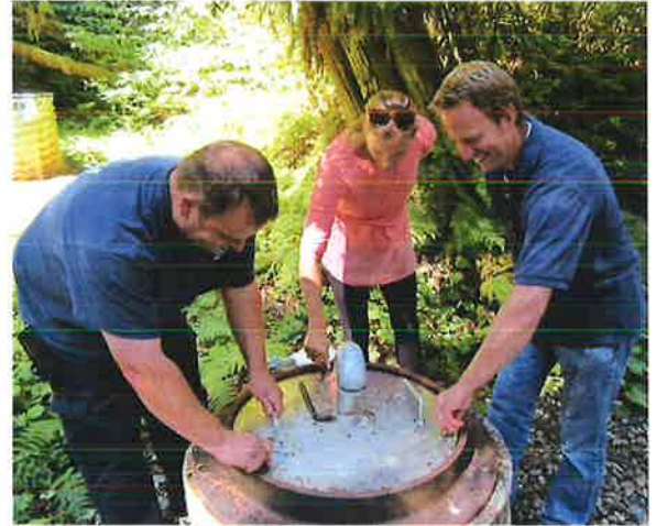
Staff at Marysville Utilities, (from left) Billy Gilbert, Kari Chennault, and Brad Zahnow, open and inspect a spring collector to ensure there are no sanitary defects.
