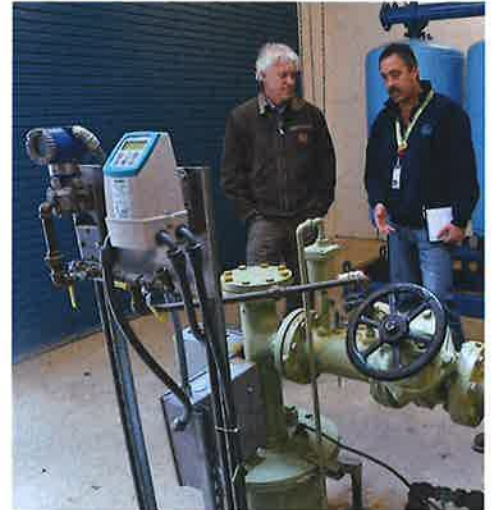
Sammamish Plateau Water Superintendent, John Anderson (right), explains why air/vacuum release valves need screening material on discharge piping during a recent visit with Derek Pell from our Northwest Regional Office.
