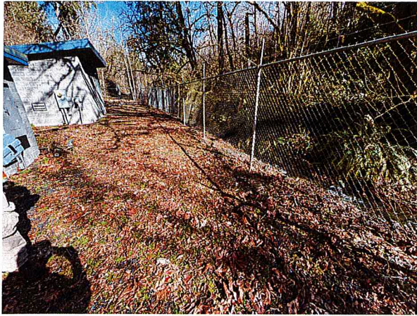
Eureka #1 Well House and Seasonal Creek
